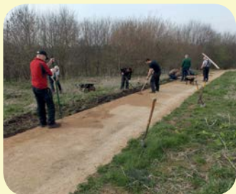
Repairing path surfaces
